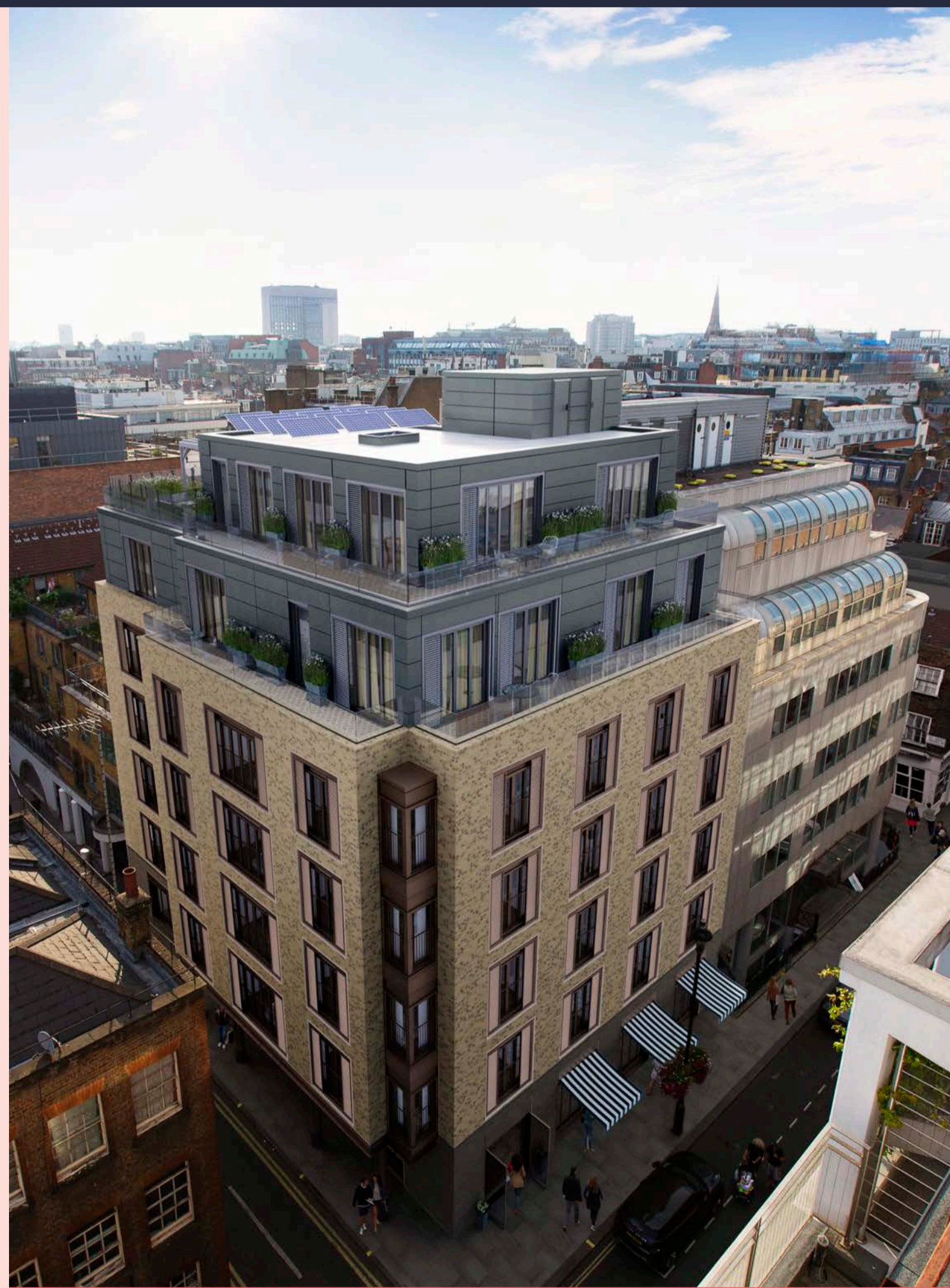
81 Dean Street & 3 Richmond Buildings
